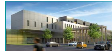
Construction of Gien (MSO GDS) € 21.4 mn
