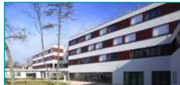
Construction of Villemomble (NH Medica) € 15.2 mn
