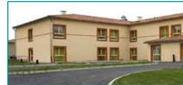
Construction of Castera (NH Medica) € 8.7 mn
