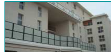
Construction of La Roche:Yon (NH Medica) € 12.2 mn
