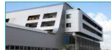
Construction of Le Havre (MSO GDS) € 75.5 mn
